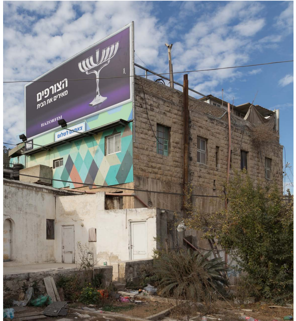
Eastern & Northern Facade Photo: Tai Pinchevsky
