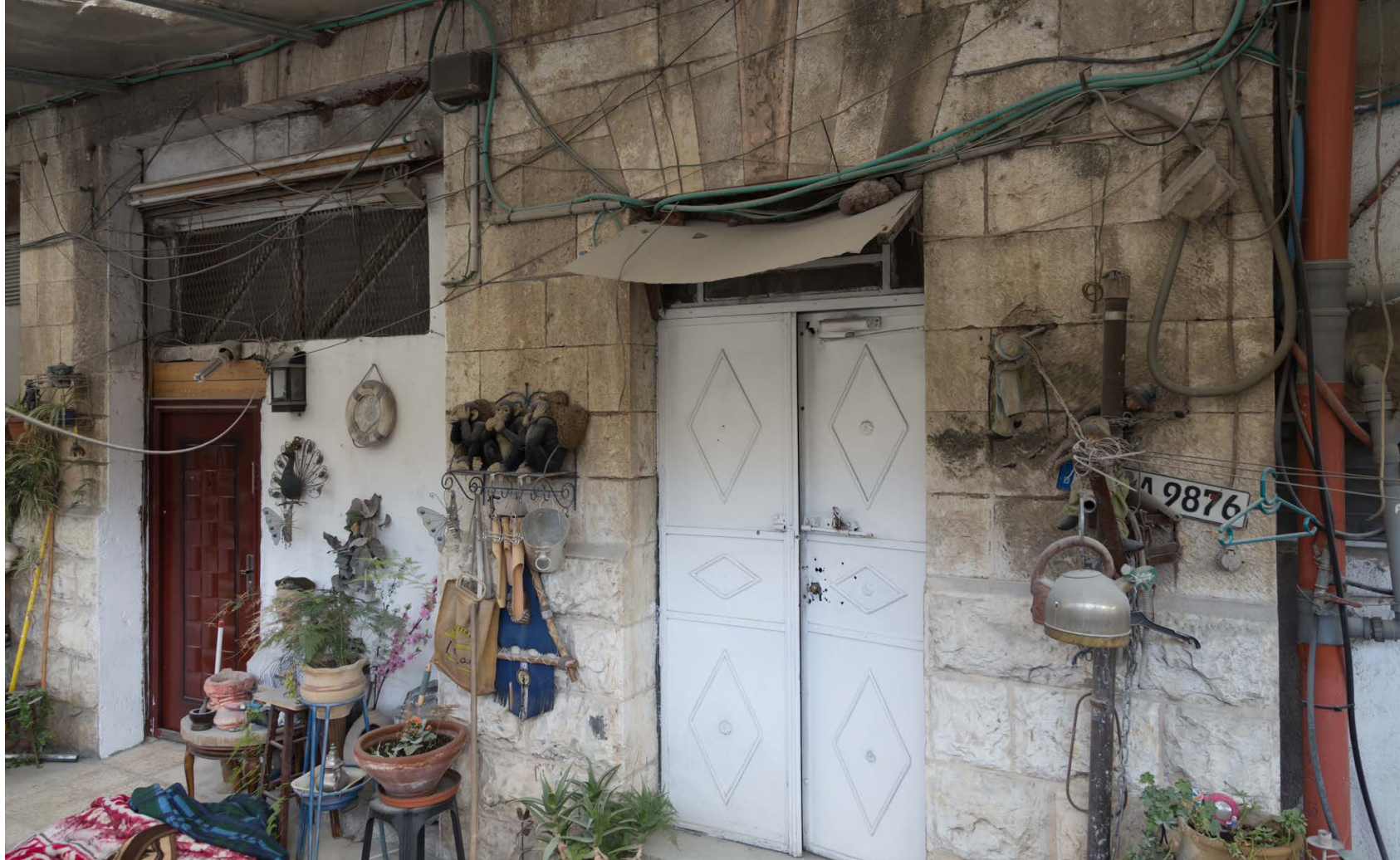
Openings on Southern Facade
