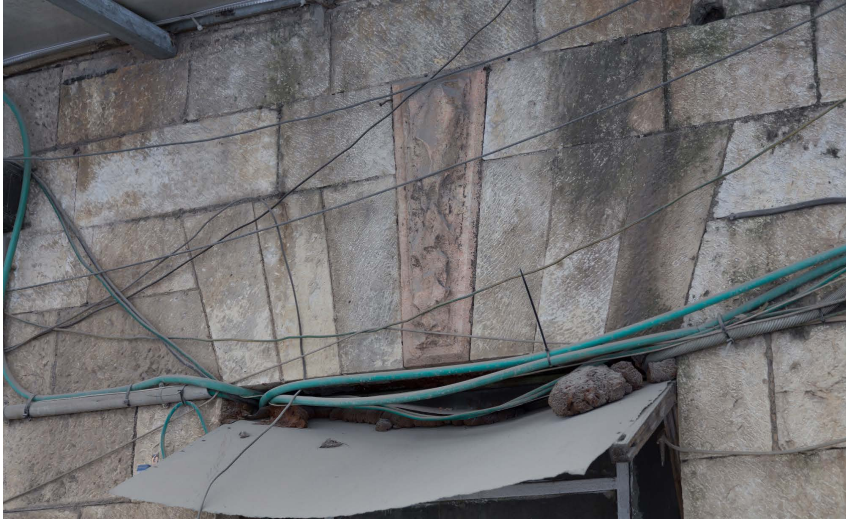
Detail on Main Entrance at the Southern Facade
