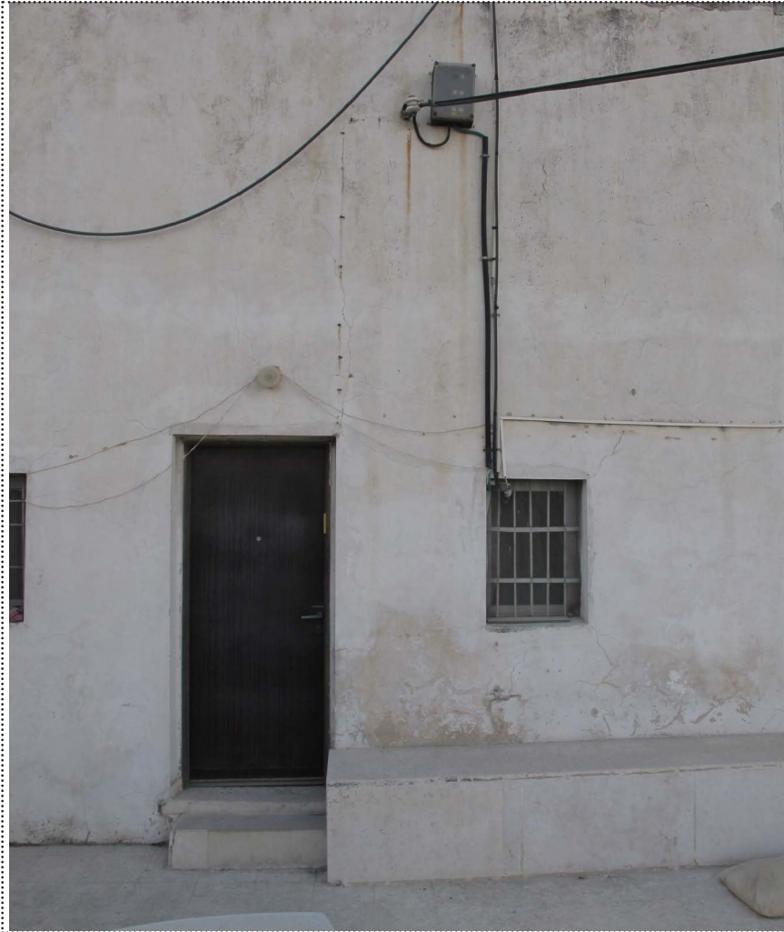
Detail Facade Photo:Hadar Porat
