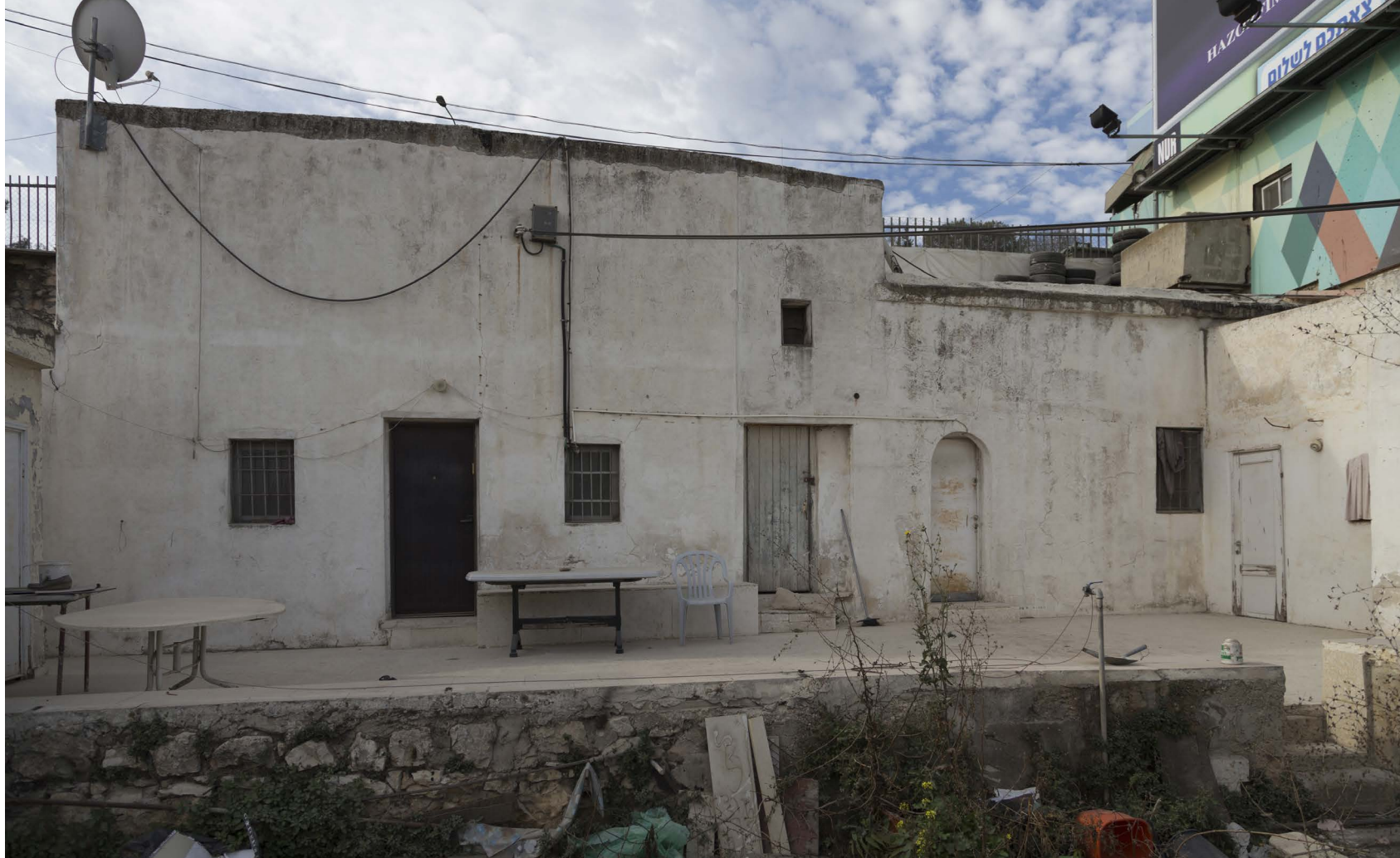
Eastern & Northern Facade
