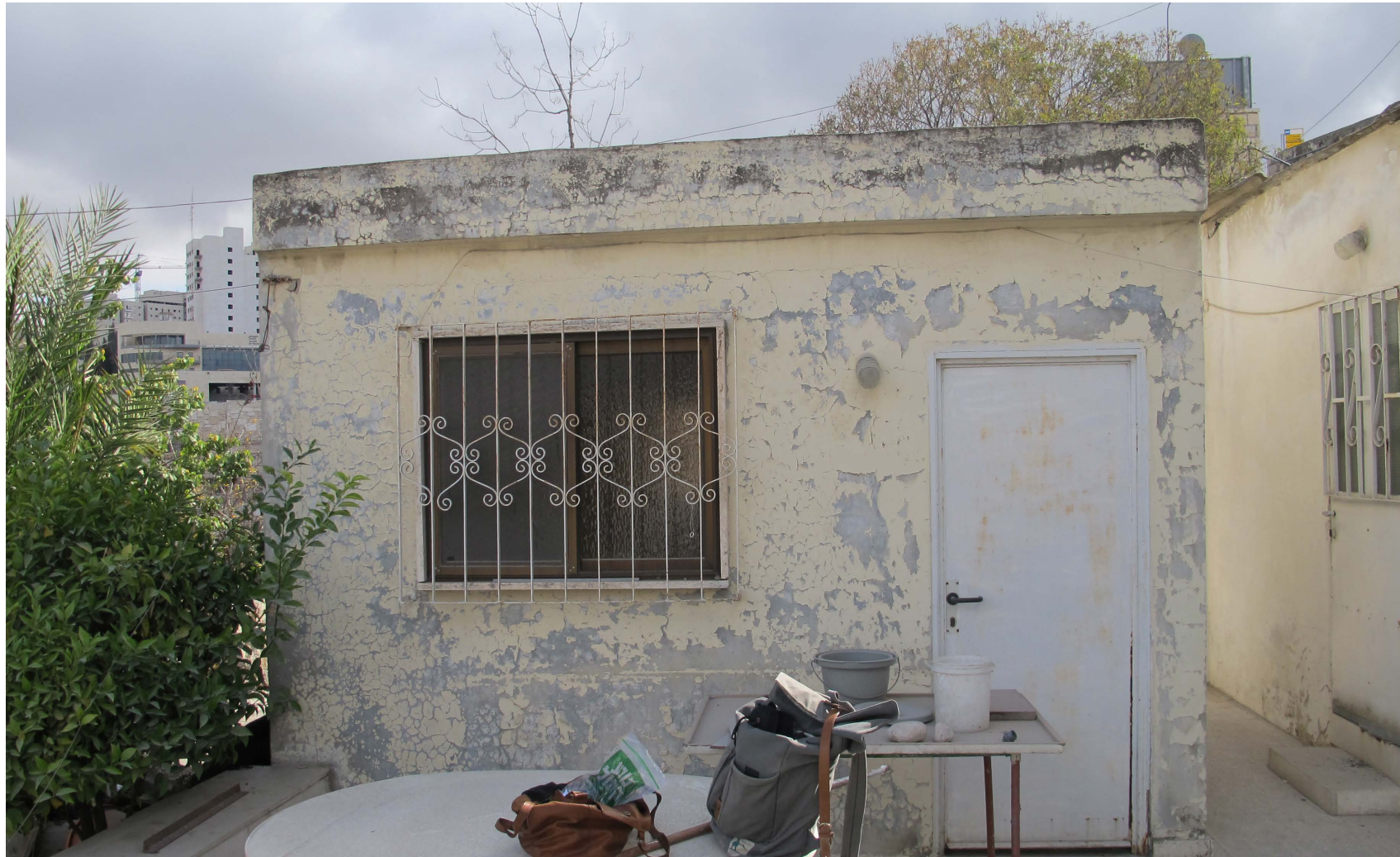
Inner Western Facade
