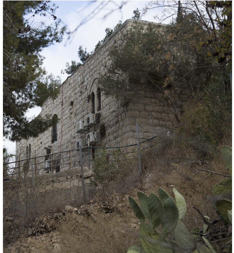
Southern Facade Photo: Tai Pinchevsky
