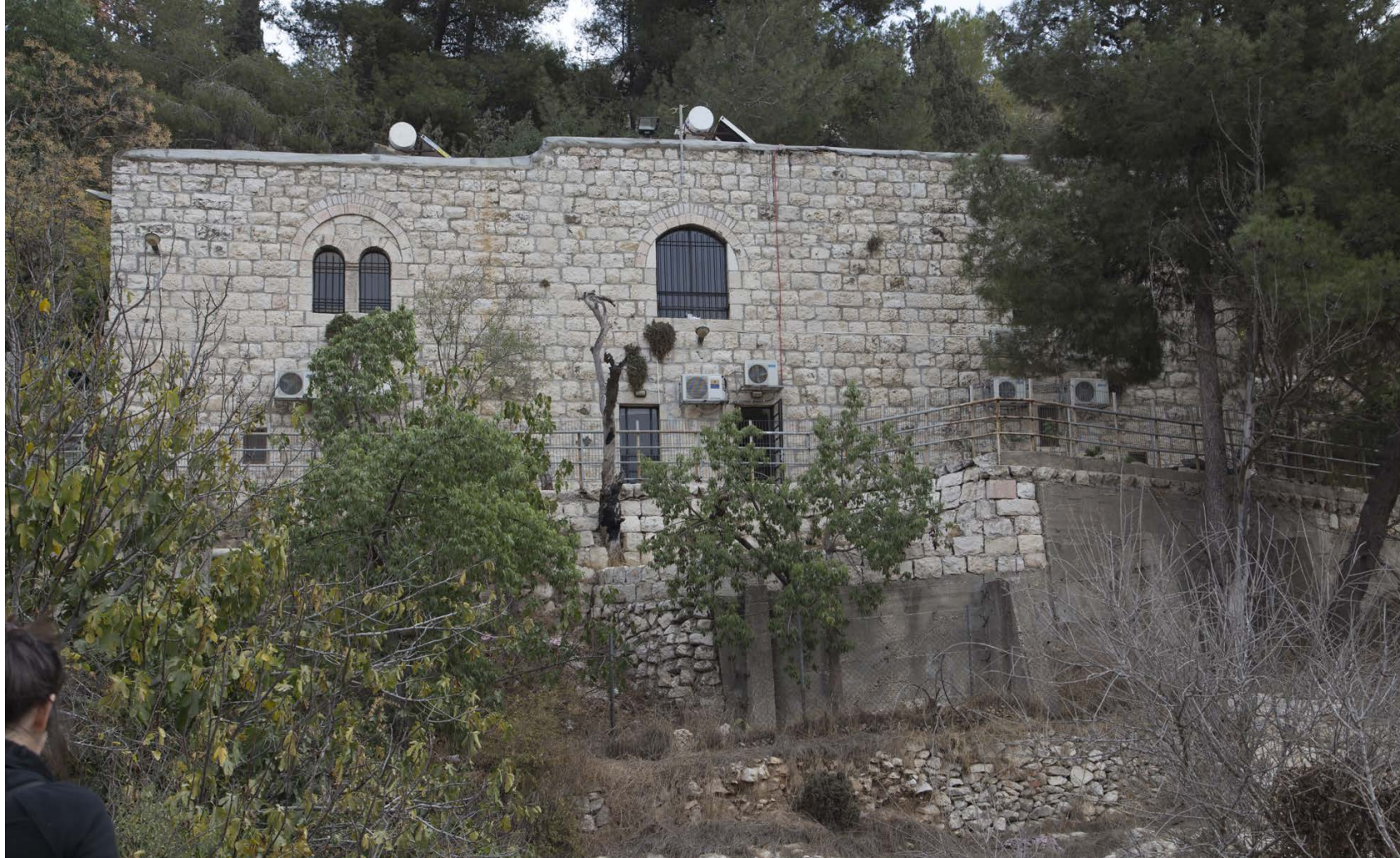
Western Facade Photo: Tai Pinchevsky
